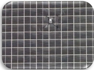
Solar farm Inspection
